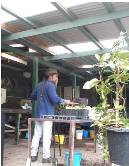
New potting roof shed keeps potters cool and dry – thanks to Max Smith.
