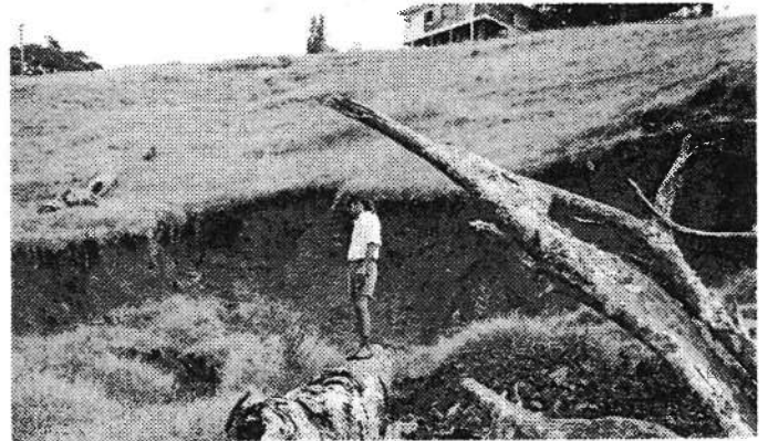
Marc Russell inspects one of the many recent slips on the Range.
