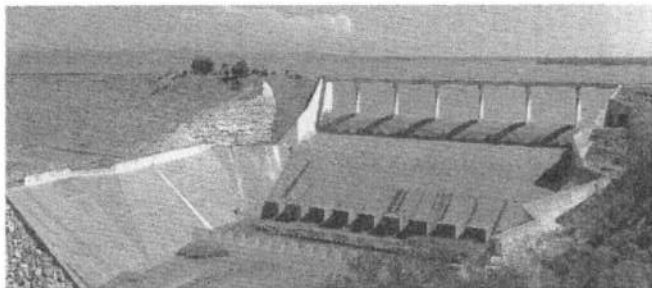
Fairbairn Dam stores water for irrigation and for the town supply of Emerald.
