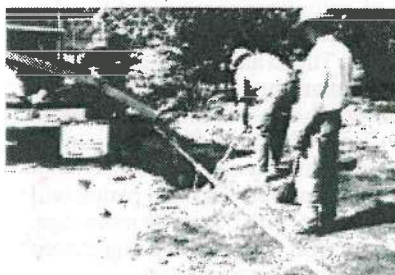
Laying more foundations...
