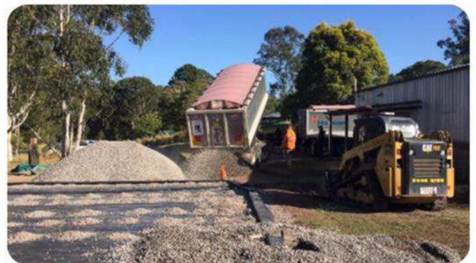
Construction of new nursery pad
