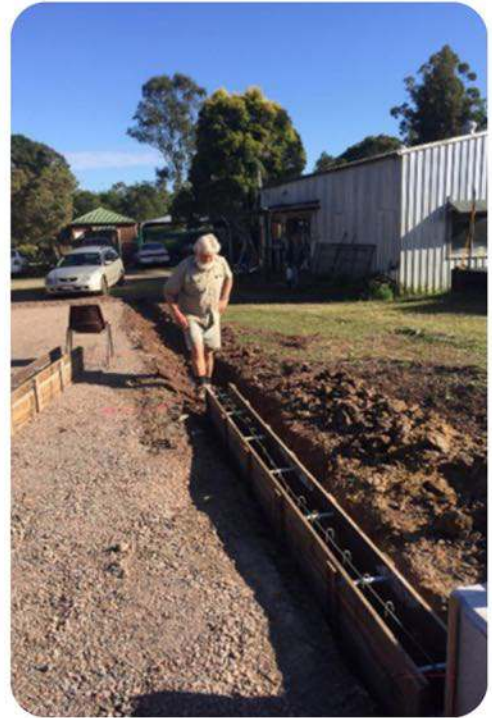
Construction underway at the Barung nursery with Wayne
