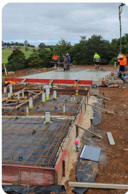
Construction underway at the new Barung nursery, 2022
