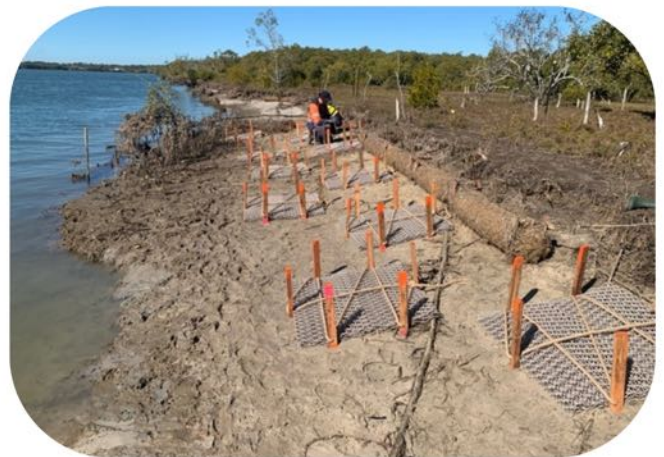
Installed BESE-Elements® Grids in River Bank (Photo – Angus Frazer)
