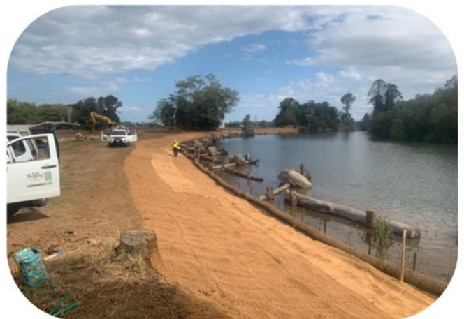
Jute mesh installed on bank for riparian planting (Photo – Angus Frazer)
